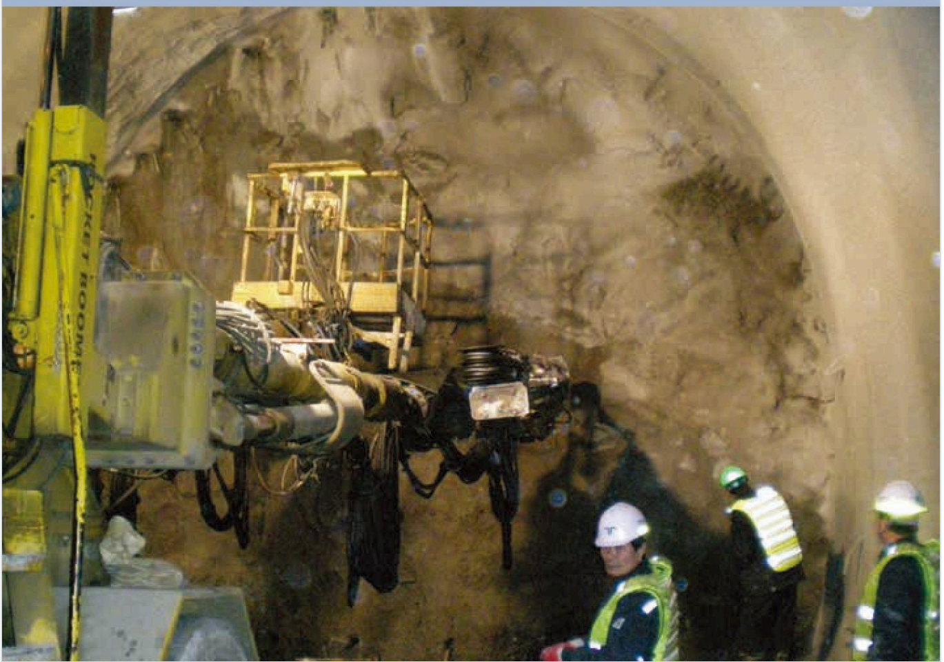
Rock bolt installation, NATM tunnel
