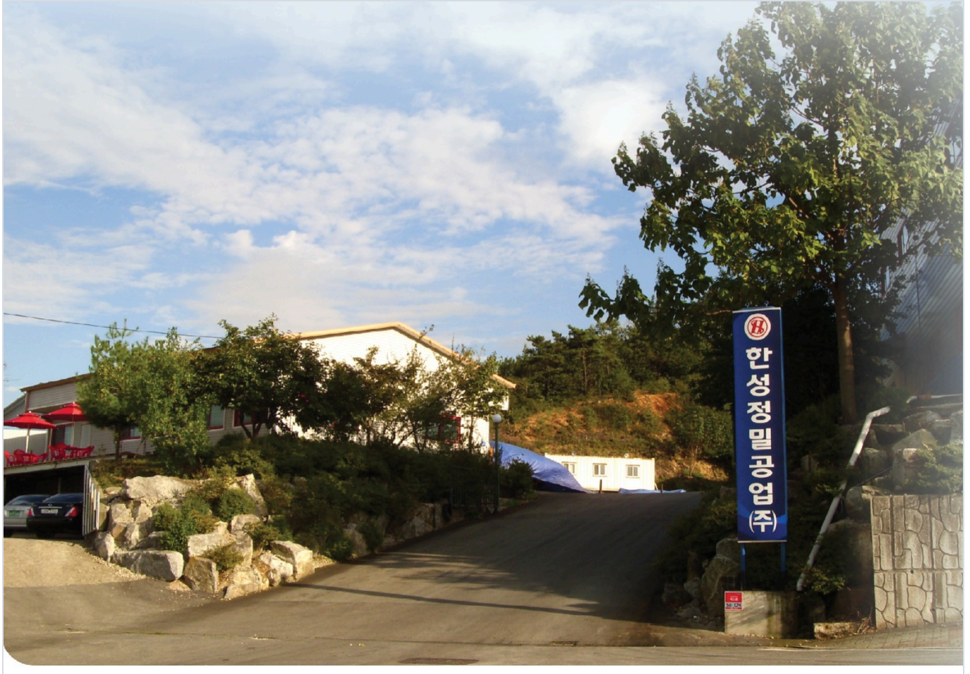
Hansung Precision plant entrance
