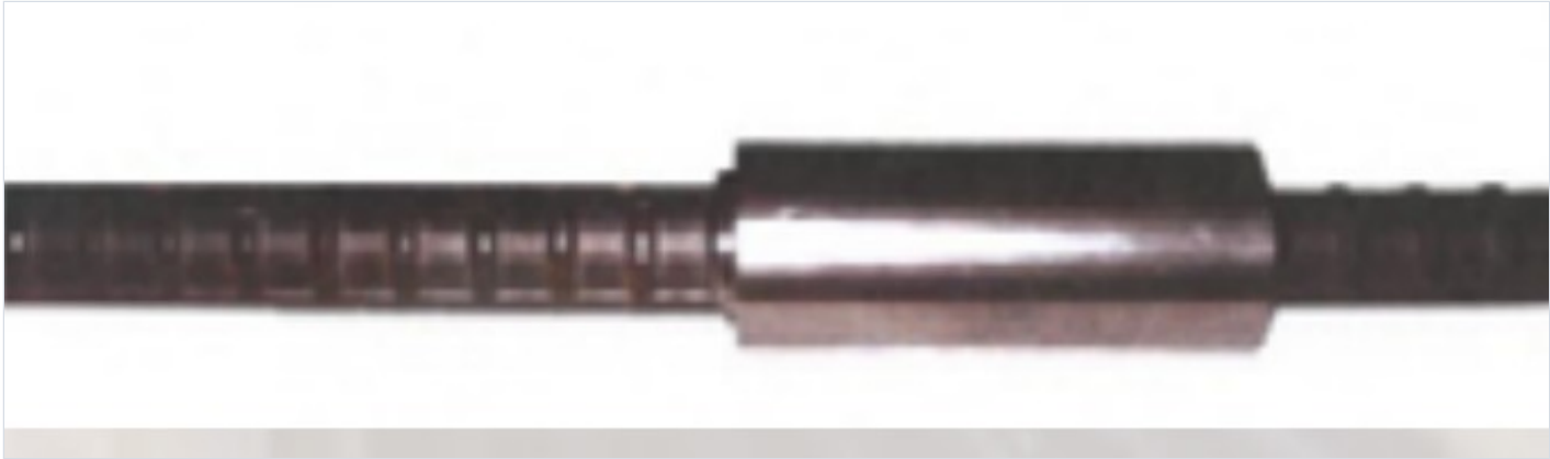
U-type field-assembly coupler
