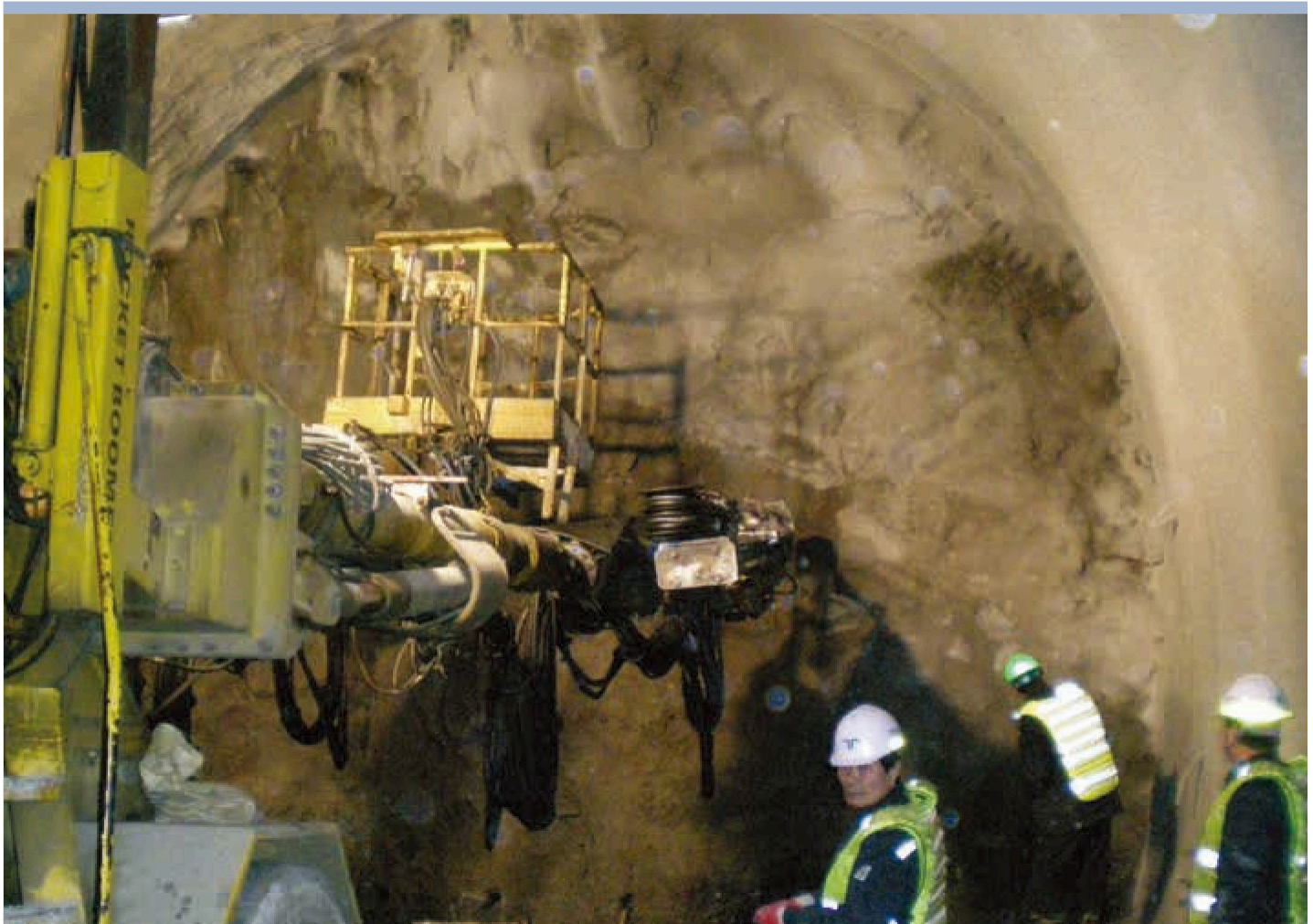
Rock bolt installation, NATM tunnel
