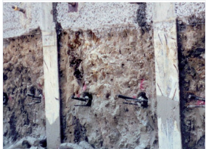
02 Face preparation before shotcrete
