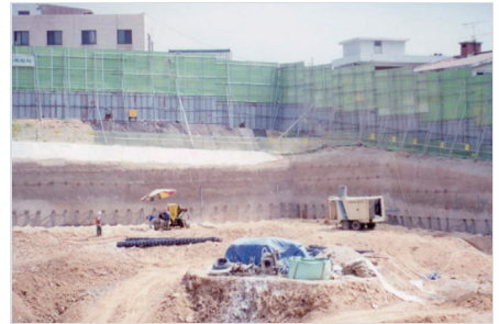
Seongsan-dong redevelopment (face prep + removable S/N + shotcrete)
