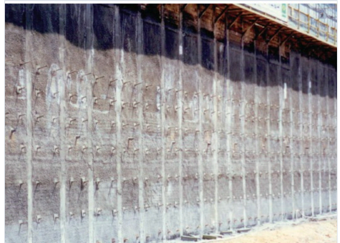
04 Retaining wall complete
